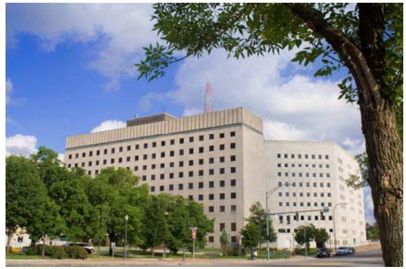
Monroe County Public Safety Building
